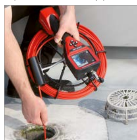
Inspection of rain downpipes
