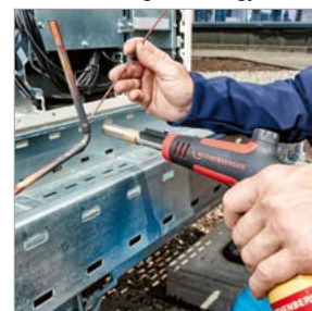
Brazing in refrigeration / air-conditioning technology
